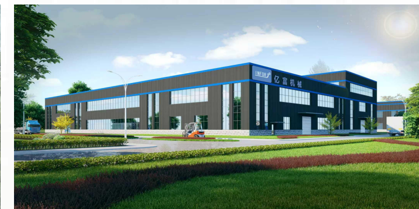
Production Base, Xiangyang, Hubei Area: 70,000m 2
